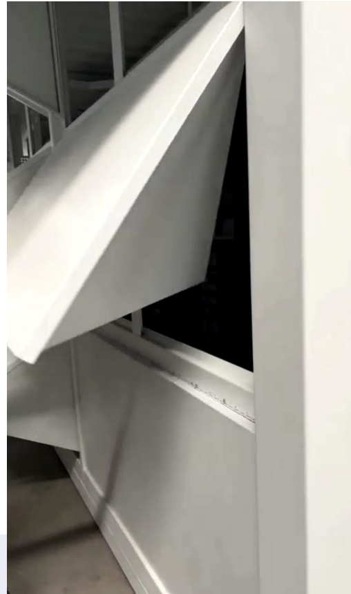
第2步: step 2: 展开支撑侧板 Unfold the support side panel
