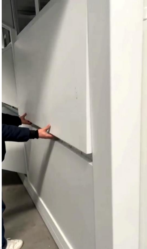
第1步: step 1: 拆卸防水进风罩固螺丝 Remove the fixing screws of the waterproof air inlet cover
